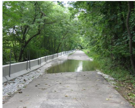
Completed concrete barriers prevented overtopping in the July 24-25, 2010, flooding along the Des Plaines River.
