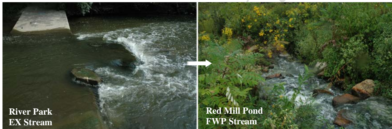
Photo 7: Concrete Stream Can Be Restored with Natural Materials to Mimic Natural Habitat Structure
