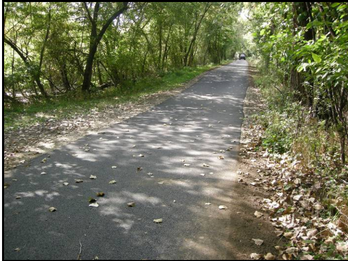
Photo 1 – Low Spot in Path Where Maintenance Crew Observed Overflow.
