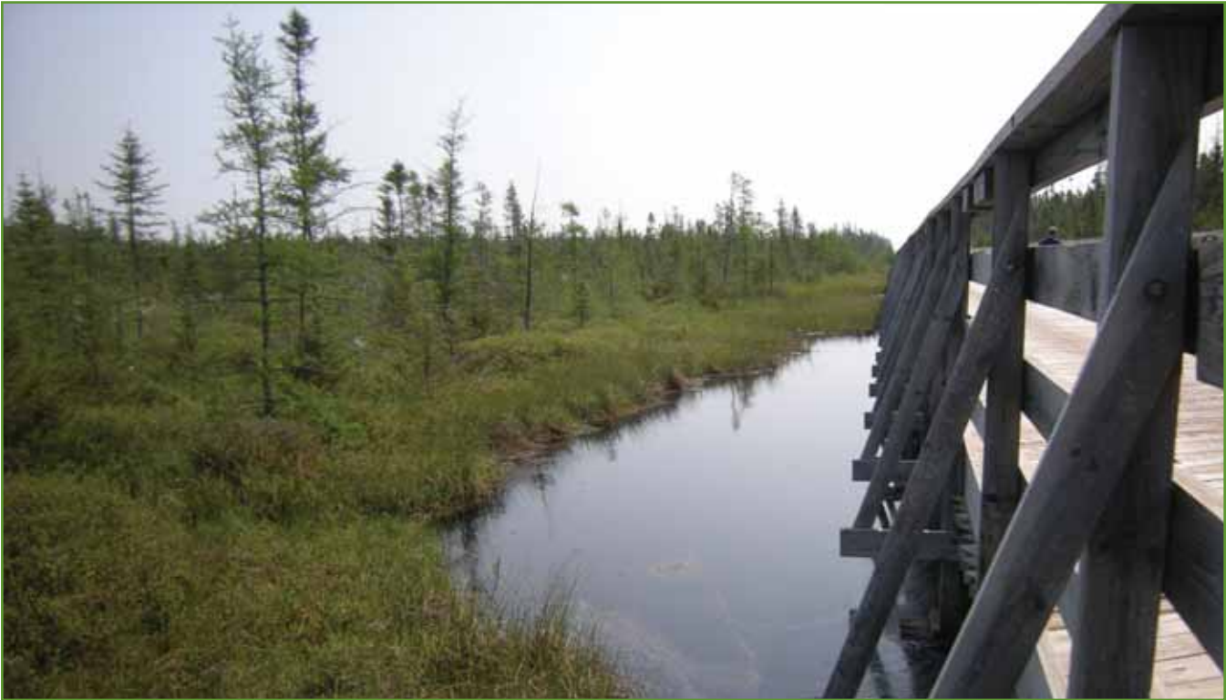
Figure 7: View of eastern end of the one quarter-mile (400 m) long bridge through swamp (aka, Bridge No. 3). Photo by USACE.
