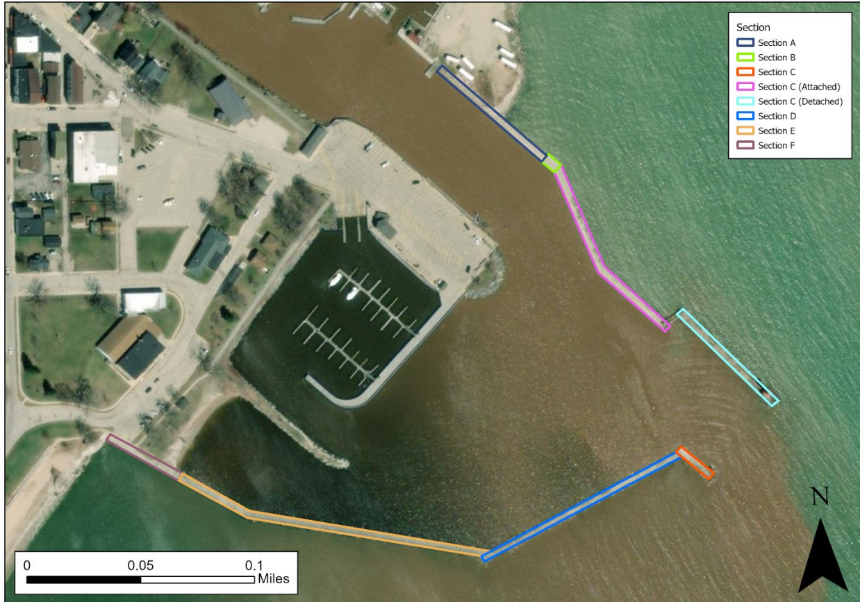
Figure 2: Aerial view of Algoma Harbor showing Sections A through F of the North Pier and South Breakwater.
