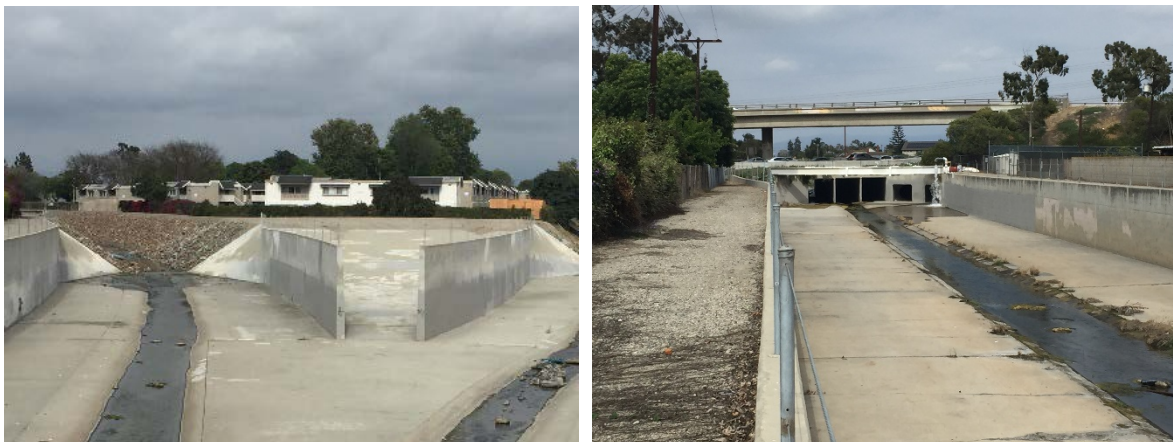
Figure 6: Reach 3 transitions from riprap lined trapezoidal (left) to concrete lined rectangular (right).
