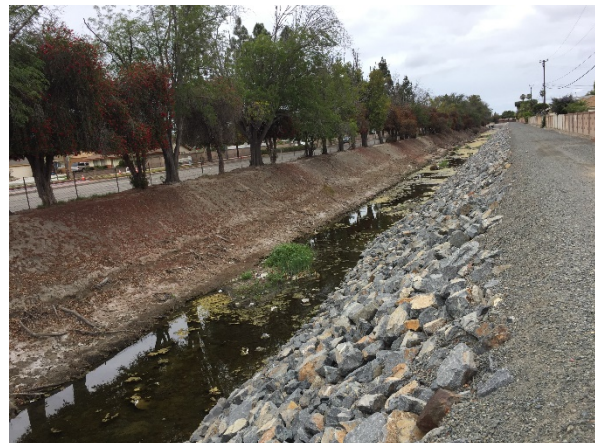
Figure 24: Reach 20 is earthen and tidally influenced downstream (left), with increased riprap applied upstream (right)
