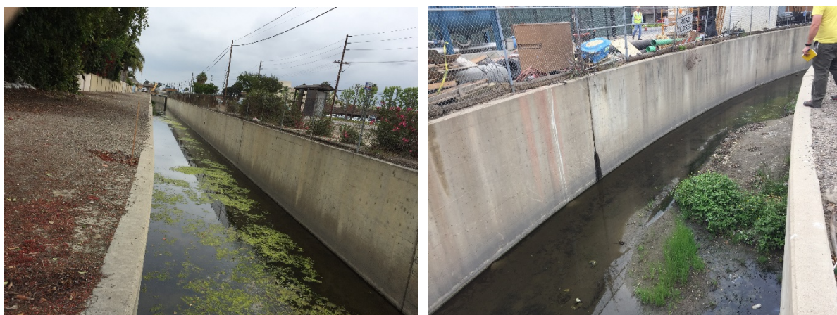
Figure 17: Reach 14 is concrete rectangular channel.
