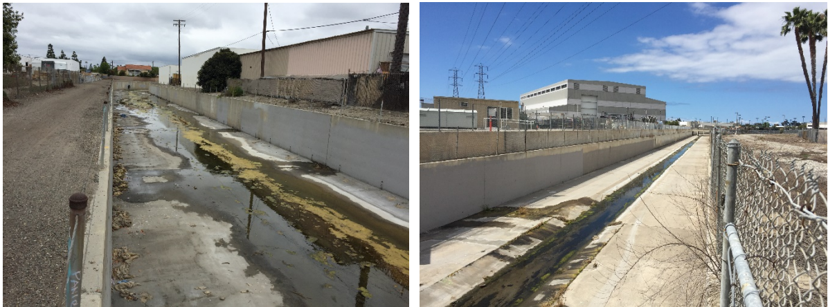
Figure 26: Reach 21 is concrete rectangular from I-405 (left) to Hazard Ave (right)
