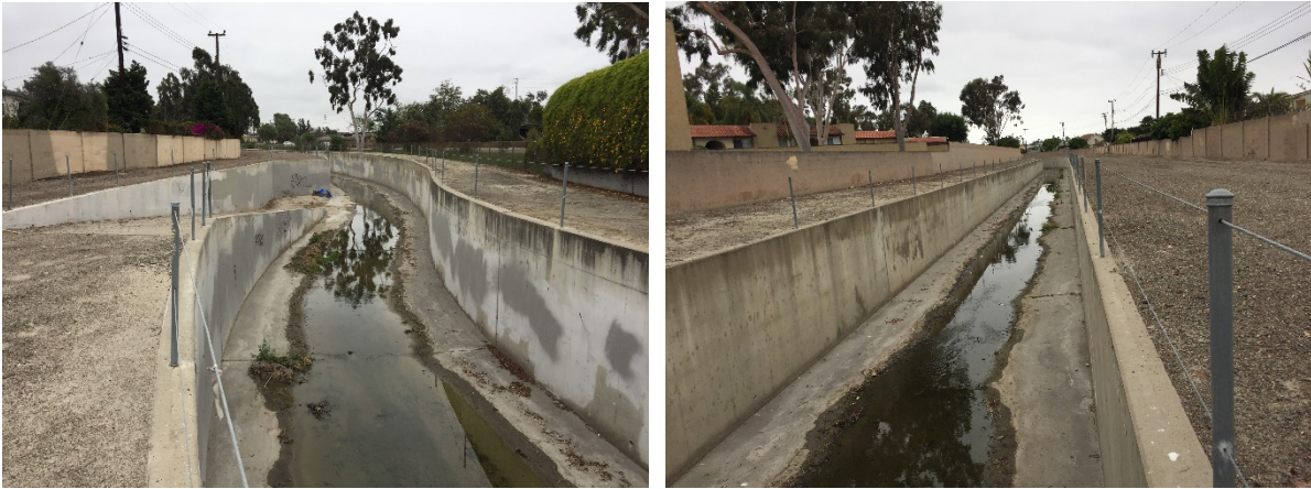
Figure 19: Reach 16 is concrete rectangular channel.
