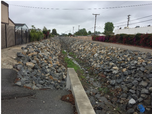
Figure 29: Reach 22 becomes riprap lined trapezoidal from Brookhurst St to Westminster Blvd.
