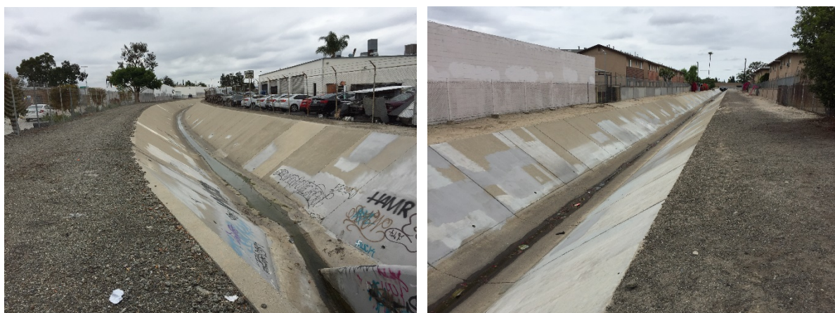
Figure 12: Reach 9 is concrete lined trapezoidal channel.
