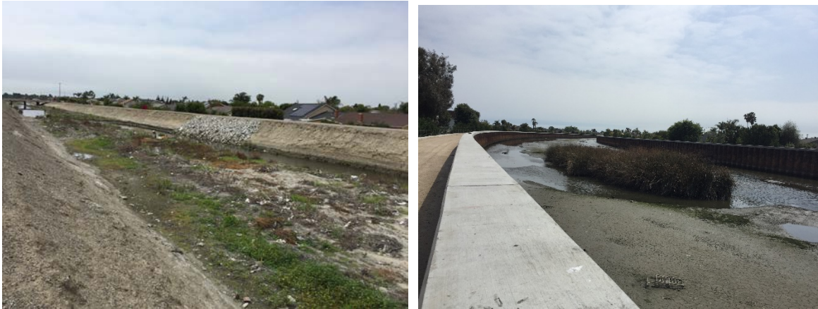
Figure 4: Reach 1 is a soft-bottom leveed reach. Recent and ongoing work has started the process of replacing earthen levees (left) with steel sheet pile walls (right).
