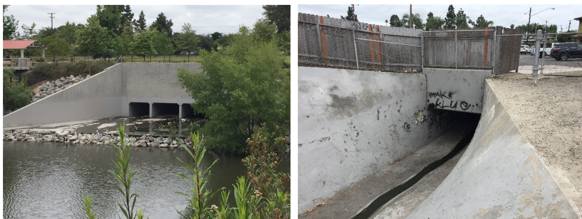
Figure 14: Reach 11 is concrete rectangular conduit that daylights at the inlet to Haster Basin.
