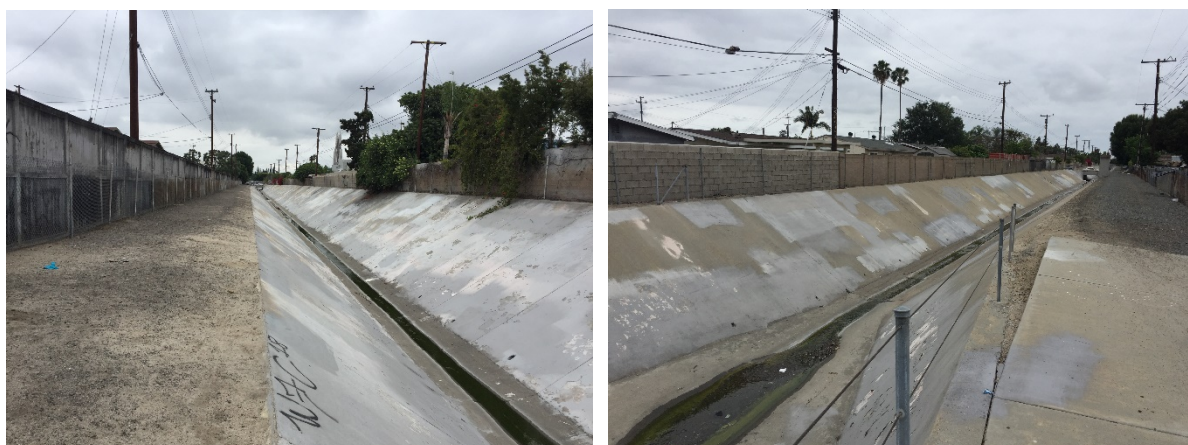
Figure 15: Reach 12 is predominantly concrete lined trapezoidal channel.
