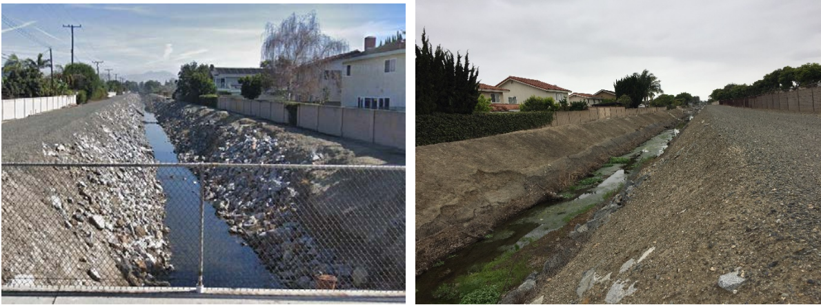
Figure 20: Reach 17 transitions from riprap lining downstream (left) to earthen channel further upstream (right).
