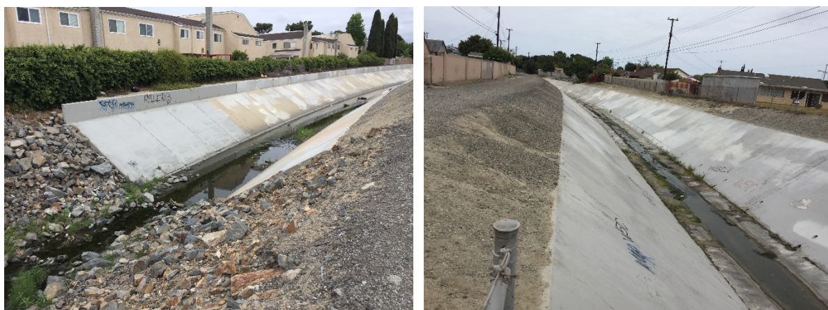
Figure 9: Reach 6 is concrete lined trapezoidal channel.
