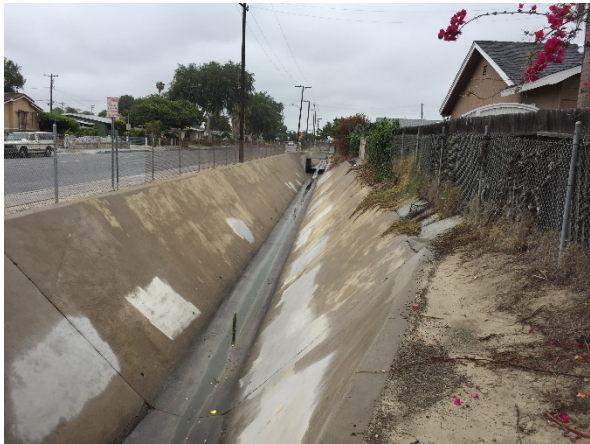
Figure 30: Reach 22 becomes concrete lined trapezoidal from Westminster Blvd. to Route 22
