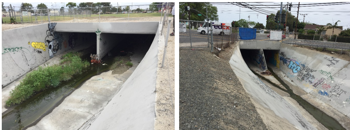
Figure 10: Reach 7 is concrete rectangular conduit that passes under Rosita Park.
