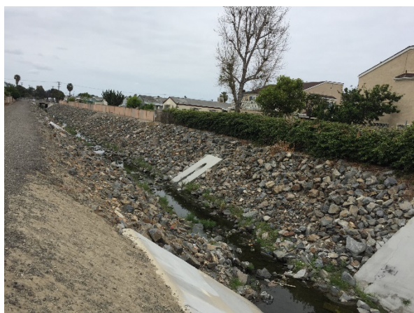
Figure 8: Reach 5 is predominantly riprap lined trapezoidal channel.
