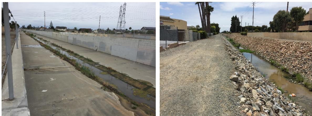
Figure 7: Concrete rectangular channel downstream (left) and riprap trapezoidal channel upstream (right) on Reach 4.
