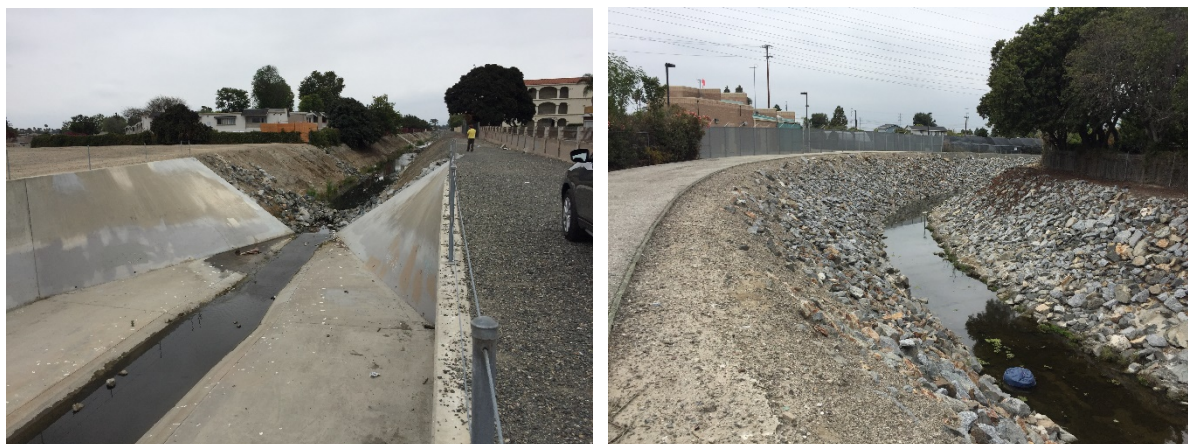
Figure 16: Earthen trapezoidal near the confluence of C05/C06 (left), transitions to riprap trapezoidal upstream (right).
