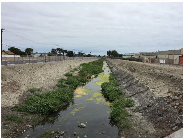
Figure 24: Reach 20 is earthen and tidally influenced downstream (left), with increased riprap applied upstream (right)
