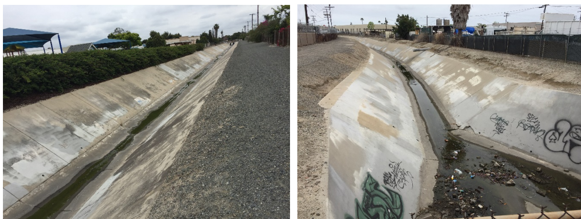
Figure 11: Reach 8 is concrete lined trapezoidal channel.
