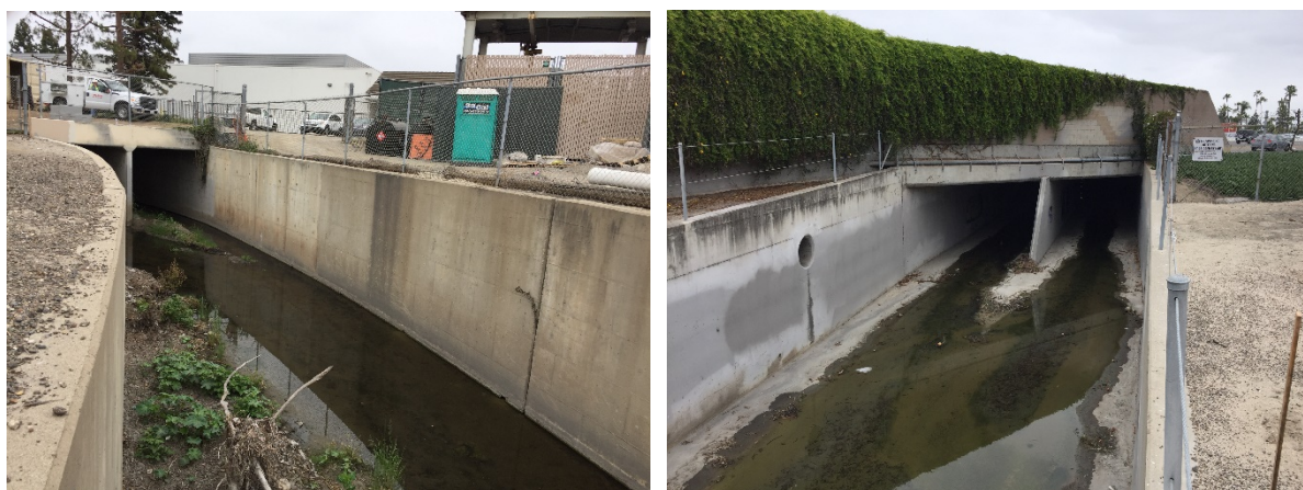
Figure 18: Reach 15 is concrete rectangular conduit from Riverbend Drive (left) to I-405 (right).
