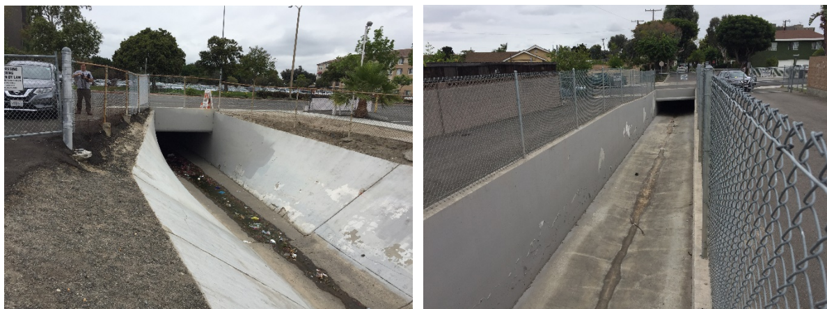
Figure 13: Reach 10 is concrete rectangular conduit that daylights just downstream of the Haster Basin outlet.
