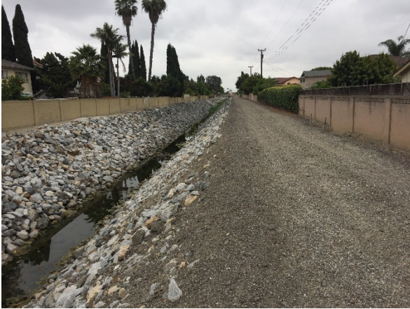
Figure 22: Reach 19 is riprap lined trapezoidal channel.
