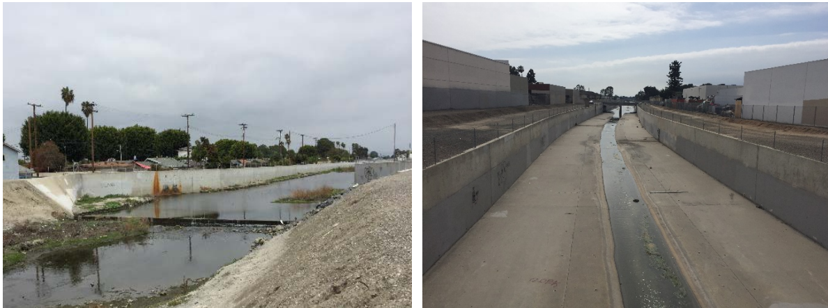
Figure 5: Reach 2 is concrete lined rectangular channel.
